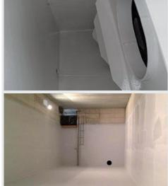
**Rivepox H**<sub>2</sub>**0** is a two-component non-toxic epoxy coating indicated for waterproofing surfaces in contact or containing drinking liquids and food thanks to the process of surface vitrification.
