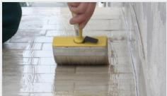
**Primer Gres** is a primer that avoids the damp rising from the ground which could compromise the sealing of a polyurethane waterproofing agent.
