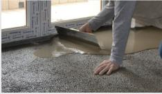
**Preparation:** the supports must be solid, consistent, well seasoned and free of removable parts, cleaned of dust, grease, oils, paints, waxes. The gypsum or anhydrite substrates as well as the prefabricated panels must be dry, compact and dust-free. Before smoothing with **Planilevel Livellina** it is essential to treat such surfaces with **PRIMER GS** beforehand. Any splits and cracks must be sealed with **Eposan**.
